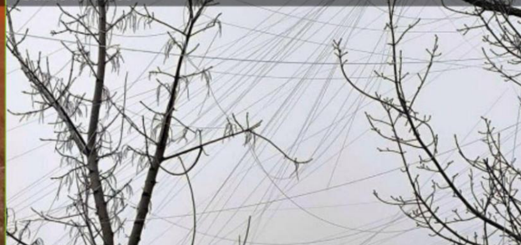
*Cable in trees*
